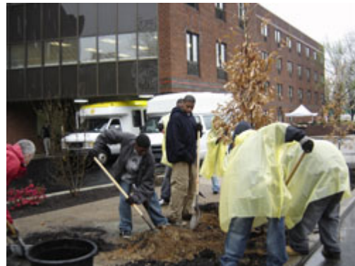
UC Green organized volunteers to transform the exterior of the LIFE location.
